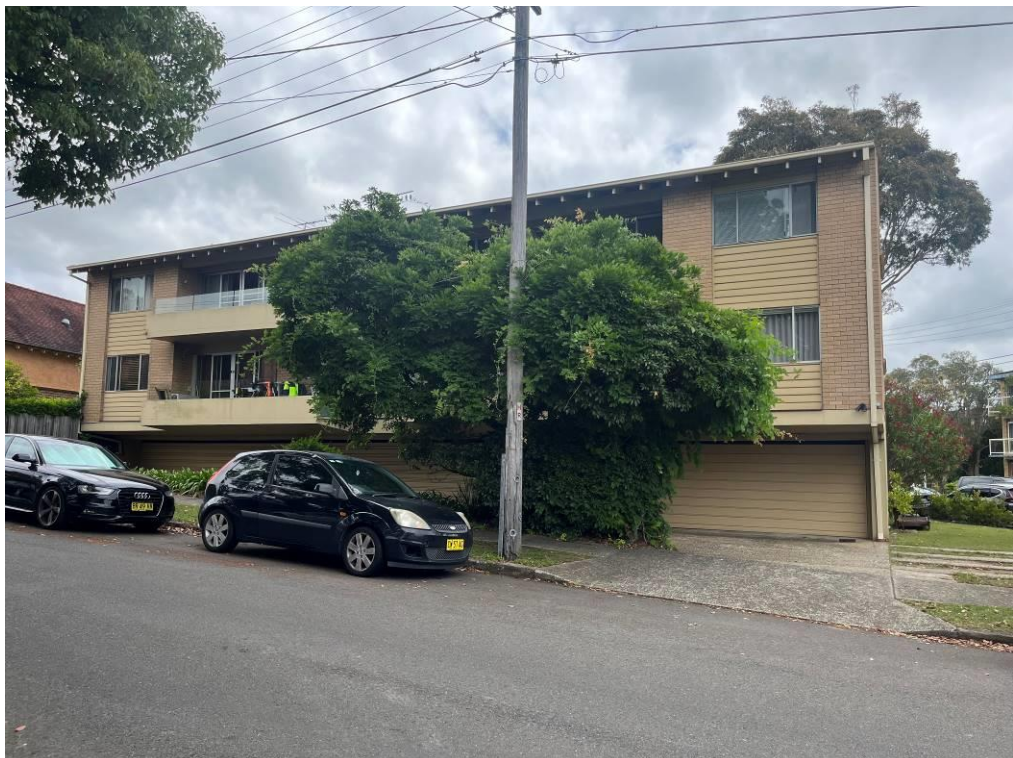
(View of Building)
