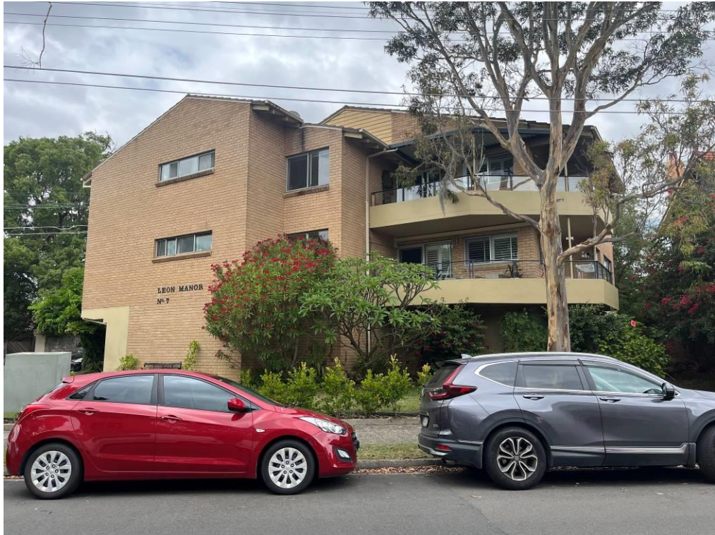
(View of Building)
